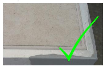
Minimum 2mm wide on each side. See that the there is a continuous joint. Shrunken silicon, projection and silicon residues on the panel are not allowed.
