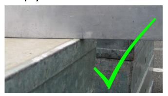
Up to a max. of 1mm allowed, in case of a newly assembled plywood no projection allowed.
