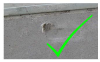
Up to the size of 2 patches D60 and a maximum depth of 1mm allowed.
