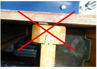
No gap allowed at screw connection of plywood.
