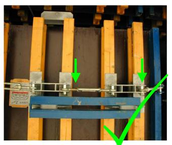
In order to guarantee that the direction of rotation of all turnbuckles is equal, the yellow screw, which additionally is marked by an "L", must be on the left side.
