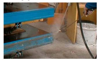
The profiles and the plywood are spread filmy with releasing agent.
