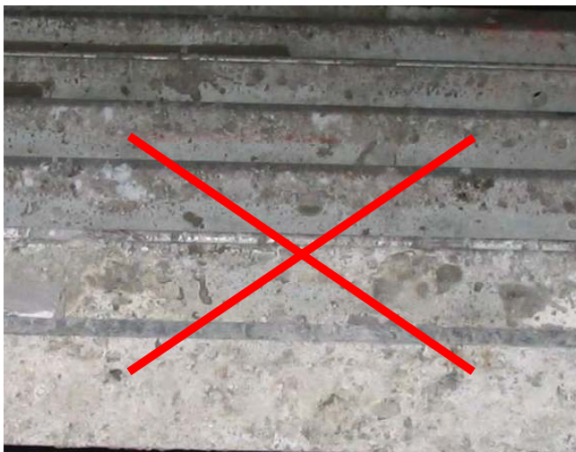
Too strong soiling at the rear side of the element frame.
