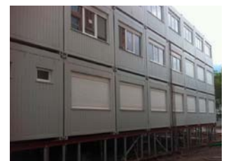
Multi-level container constructions
