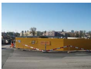
Construction site fences
