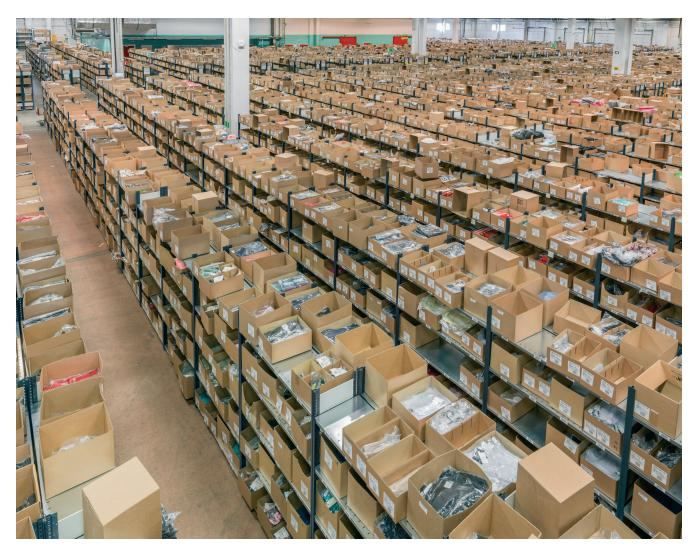
EAB's shelving stands extremely stable - moving neither sideways nor backwards and forwards. The secret lies in the intelligent design of both uprights as well as ends and shelves: bracket plates stabilise the ends through the underframe. Ingenious shelf clips fix the shelf in the correct position. And box profiles that are movable lengthways provide bearing capacity as well as a degree of flexibility in the shelving.
