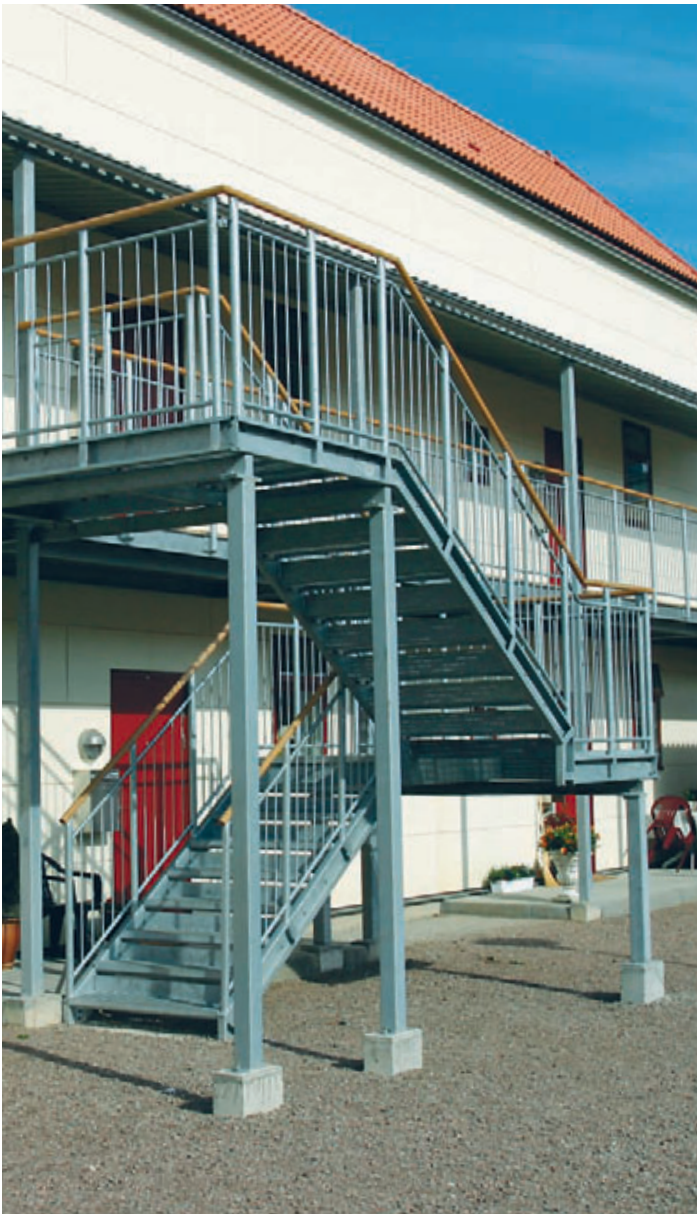
Staircase with steel plate treads covered with tiles, child-proof balustrade and wooden handrail.
