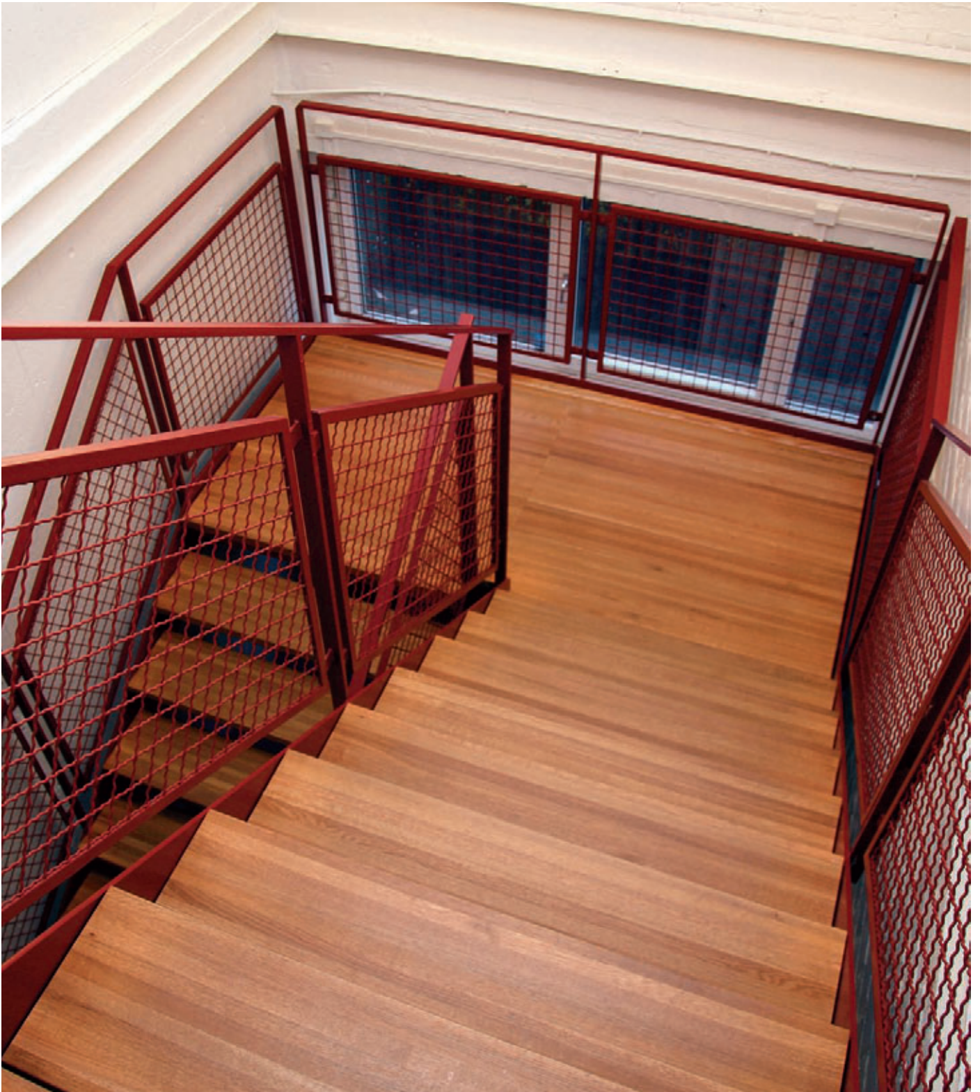
Staircase with wooden treads and Special balustrade.
