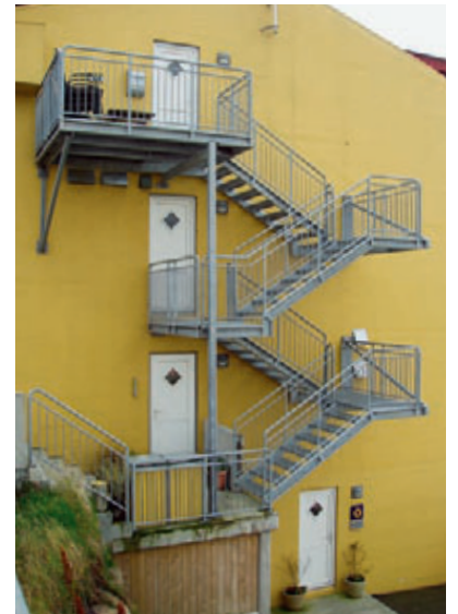
Multi-flight staircase with different types of fixings.
