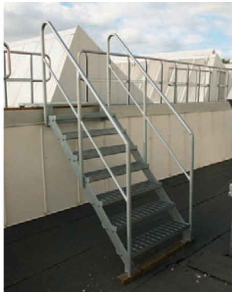
Staircase with stringer of WUC-profile.
