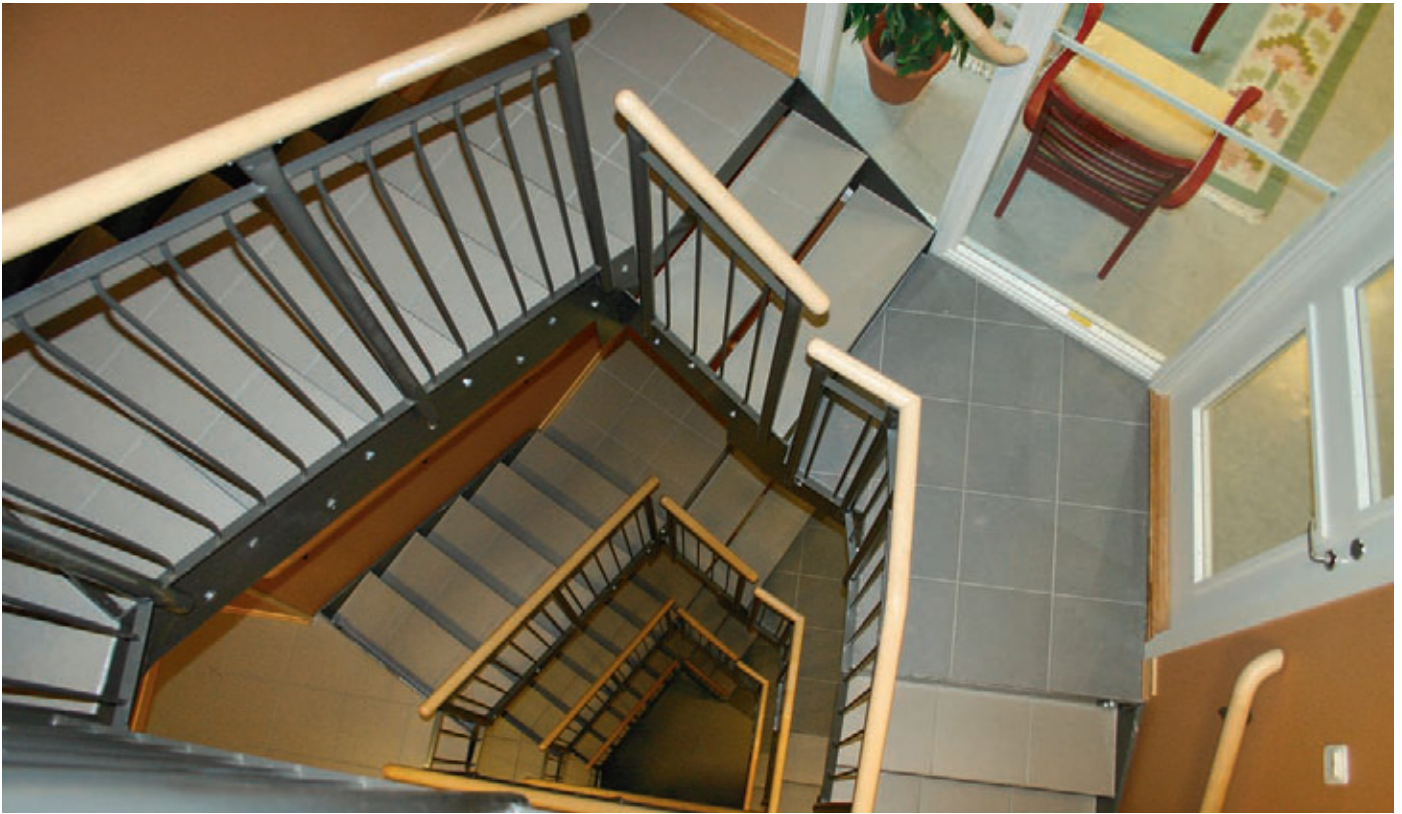
Staircase with steel plate treads covered with tiles, child-proof balustrade and wooden handrail.
