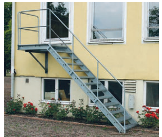
Straight flight staircase with landing and bracket.
