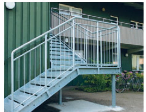
Staircase with Child-proof Balustrade.
