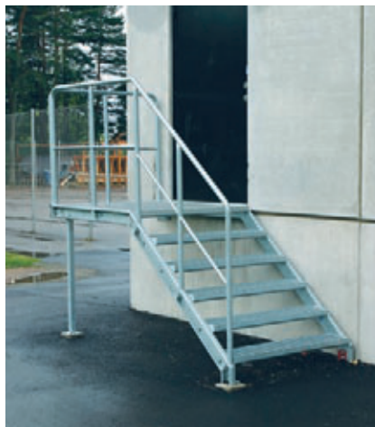
Staircase with support leg.
