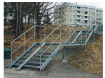
Staircase with pram-ramp.
