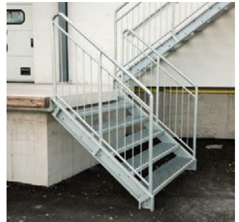
Staircase with stringer of WUC-profile.
