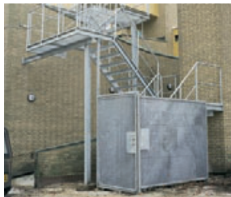
Escape staircase with protective cage.
