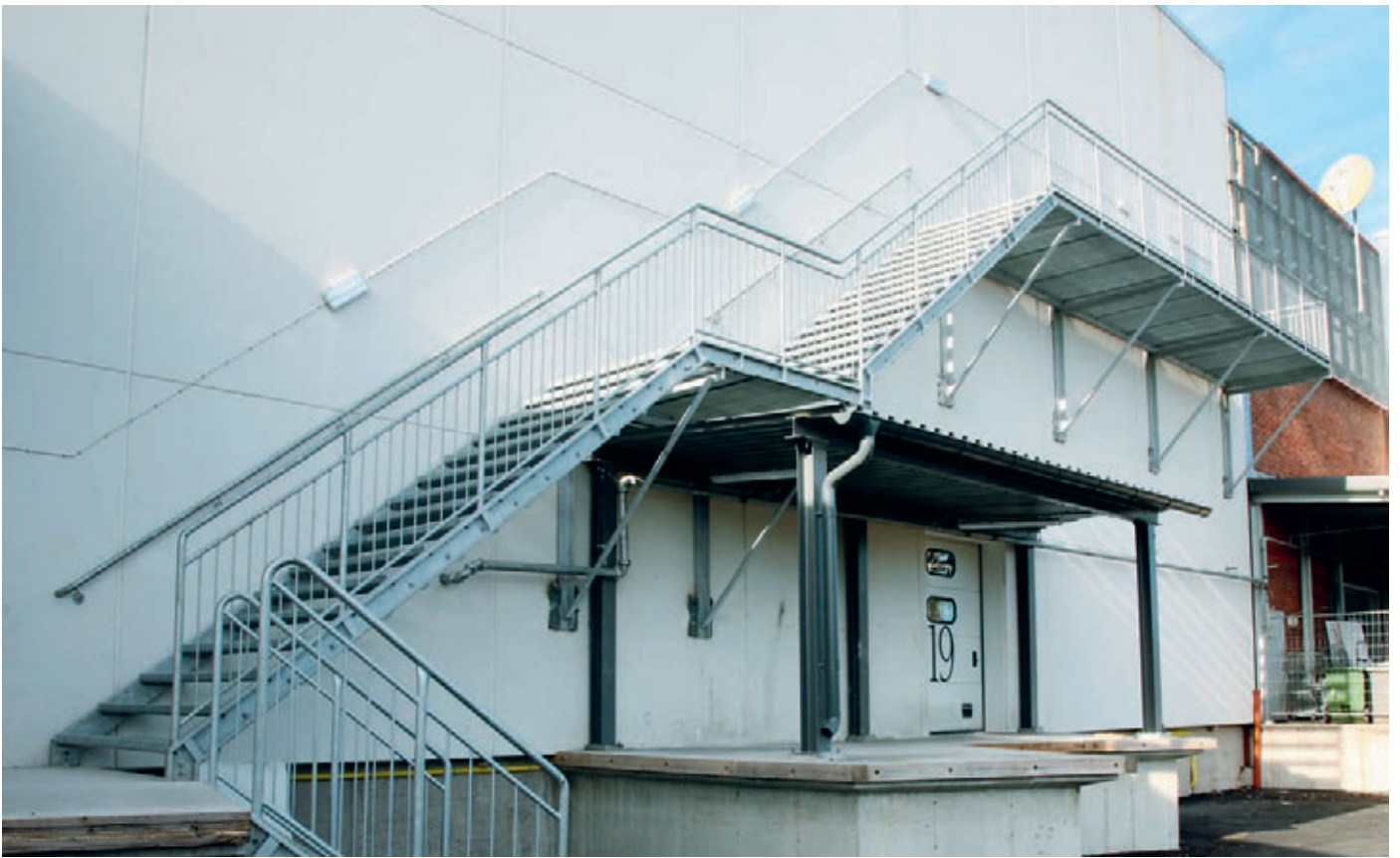
Multi-flight staircase with Child-proof Balustrade.
