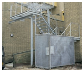
Escape staircase with protective cage.
