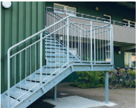
Staircase with Child-proof Balustrade.
