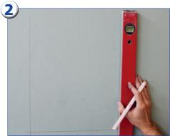
Mount installation dimension + 6 mm cut end on the desired spot. Make sure that the angle is 90°.
