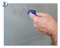
Saw out installation opening using a knife or a jigsaw. Precise working means less post-treatment afterwards.
