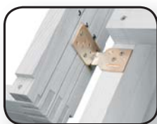
Installation on rafters
