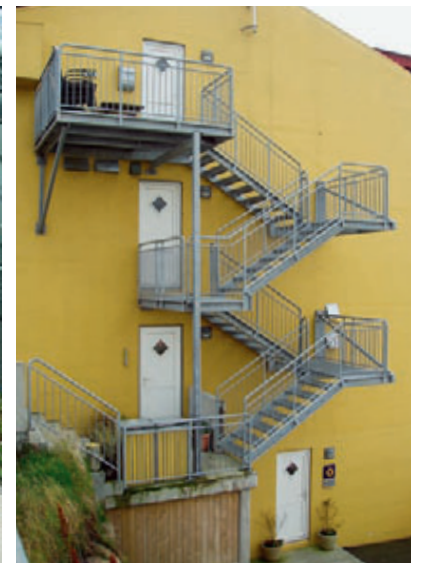
Multi-flight staircase with different types of fixings.
