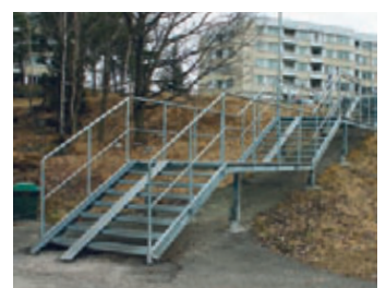
Staircase with pram-ramp.
