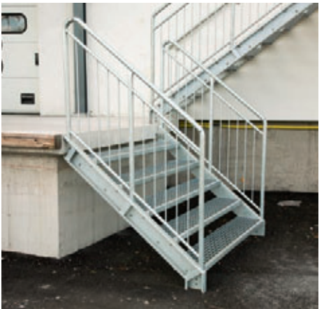
Staircase with stringer of WUC-profile.
