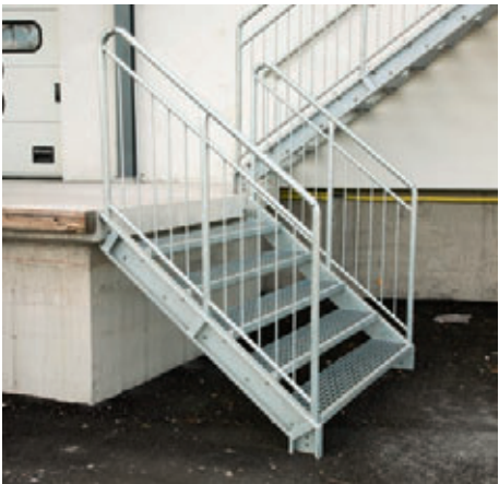
Staircase with stringer of WUC-profile.
